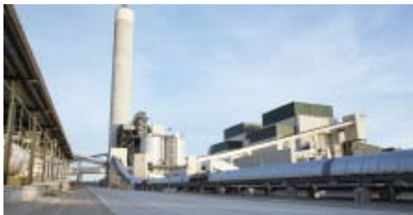
The two 800 MW supercritical, coal-fired generating units at the Prairie State Generating Company began commercial operation in Fiscal Year 2012-13.
