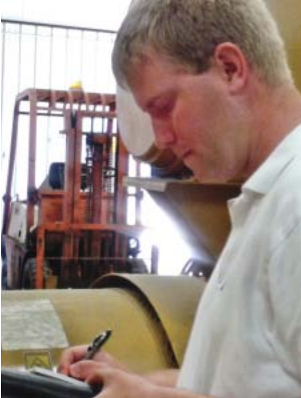
IMEA Electrical Engineer Tanner Jones checks the performance of a diesel generating unit in Sullivan, Illinois.
